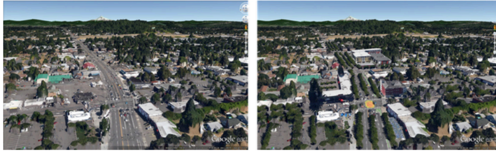
ACTIVE AND SAFE DIVISION ST. : Before and after aerials looking east along SE Division St. Retrofit includes new buildings, marketplace, community plaza, intersection painting, bike lanes, and crosswalk improvements.
